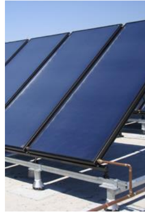
Solar panels on Metro School in Charlotte (Photo Credit: CMS)
