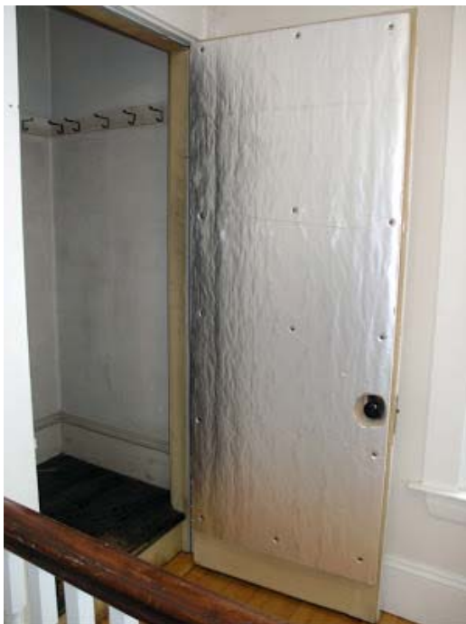
Figure 80. Insulated attic doorway
