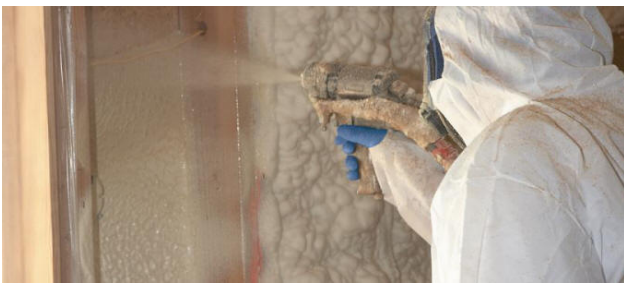
Figure 71. Spray-foam Insulation into a wood stud wall cavity
