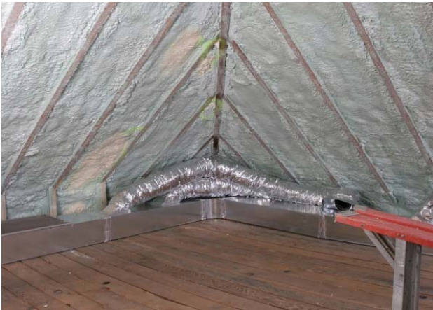
Figure 68. Air sealed attic space
