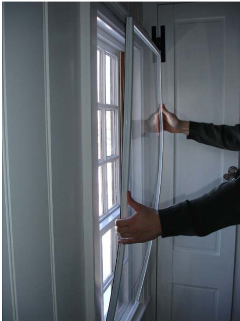
Figure 75. Internally magnetized glass pane Insert by Climate Seal.
