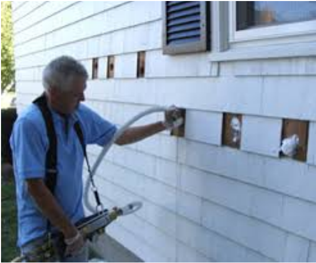
Figure 70. Injection Foam Insulation retrofit in an existing home
