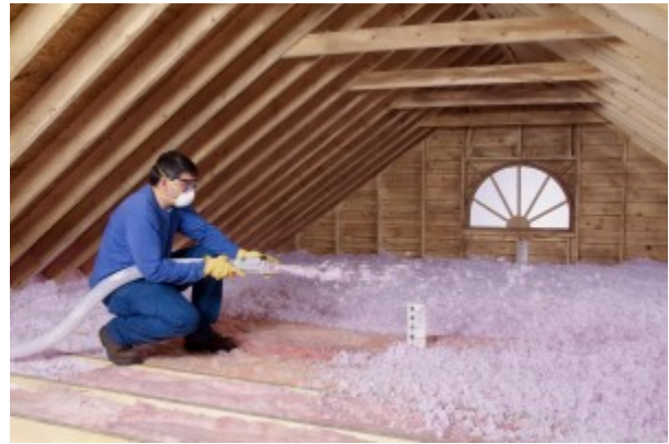
Figure 69. Addition of Blown-In attic insulation
