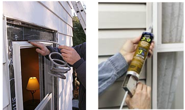
Figure 74. Foam backer rod and sealant at existing windows
