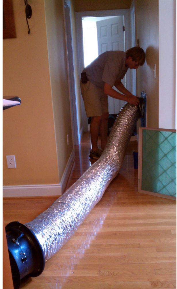
Figure 9. Duct Blaster diagnostics test underway
