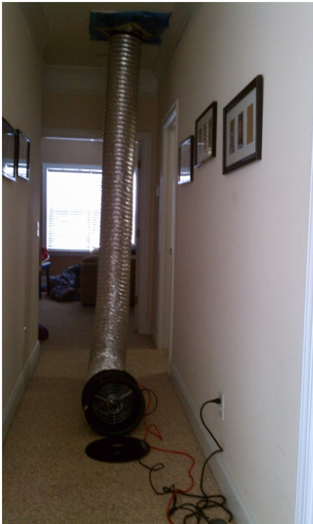
Figure 30. 'Duct Blaster' diagnostics test underway
