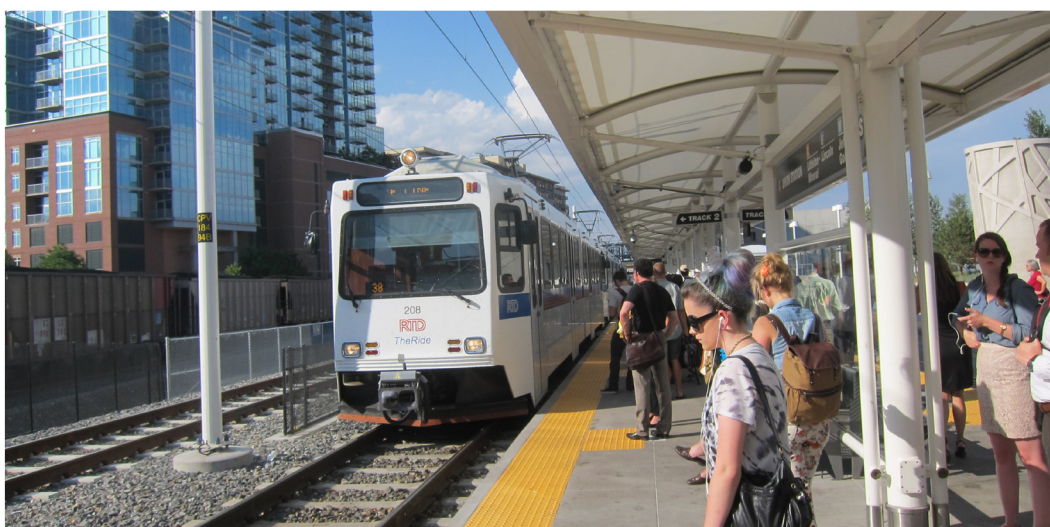
Above, Denver RTD LRT. Image Credit: Stephen Rees
